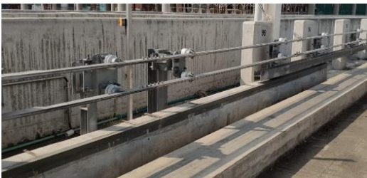
Gambar 2. Third Rail dan lintasan LRV (Light Rail Vehicle)
