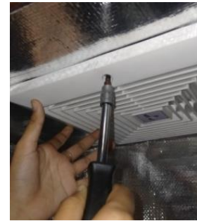
Gambar 7. Proses Pemasangan Casing Exhaust fan
