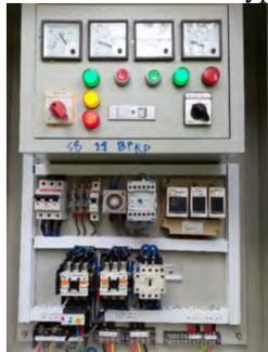
**Gambar 3 Panel Instalasi Pompa Sumur Bor**
