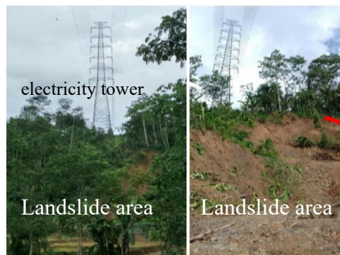
Figure 1. Landslide location under High Voltage Air Line (SUTT) electricity tower.
